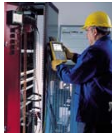
Site ALSTOM POWER Service Massy - France
